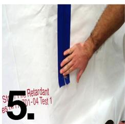
5. Once you have reached the end of the strip, remove the backing and dispose of it.
