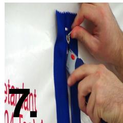
7. Once the strip is unzipped, make a perforation with a blade at the top of the desired opening.
