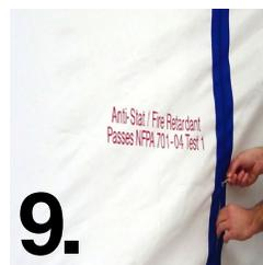
9. Once cut, press the two strips tightly onto the sheeting on both sides of the opening to ensure a secure adhesion.
