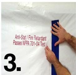
3. Once adhered, continue to lay and peel the backing off of the zippers as you place the strip onto the sheeting. Gently press it onto the sheeting as you make your way down.
