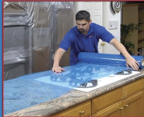
Applying Counter Top Cover™
