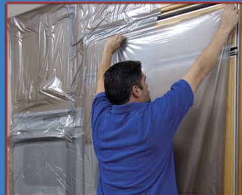
Applying Cabinet Cover™
