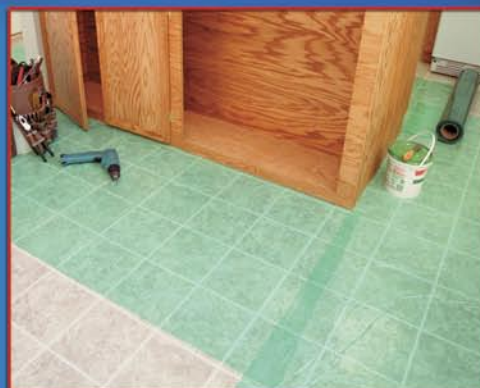
Floor Cover 45™ cut around built-in
