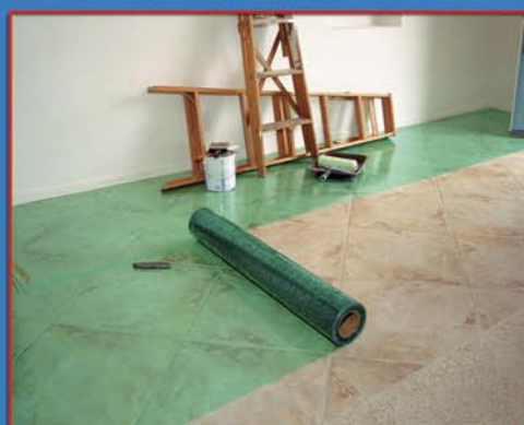
Floor Cover 45™ rolling out on Hallway
