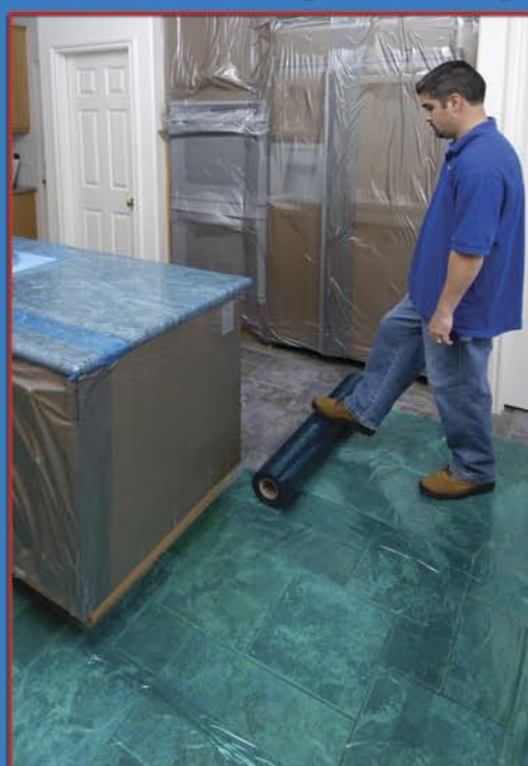
Rolling out Floor Cover 45™ in Residential Kitchen
