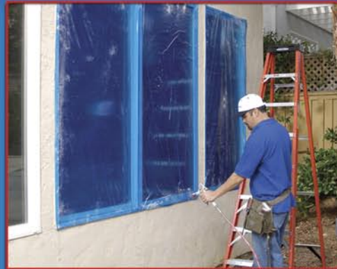
Glass being protected during stucco painting
