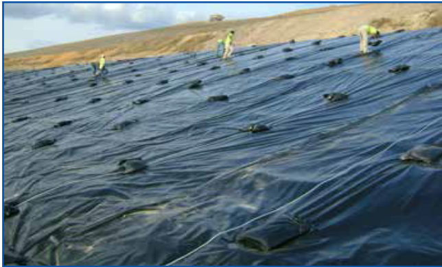
Temporary Rain Shed Cover
