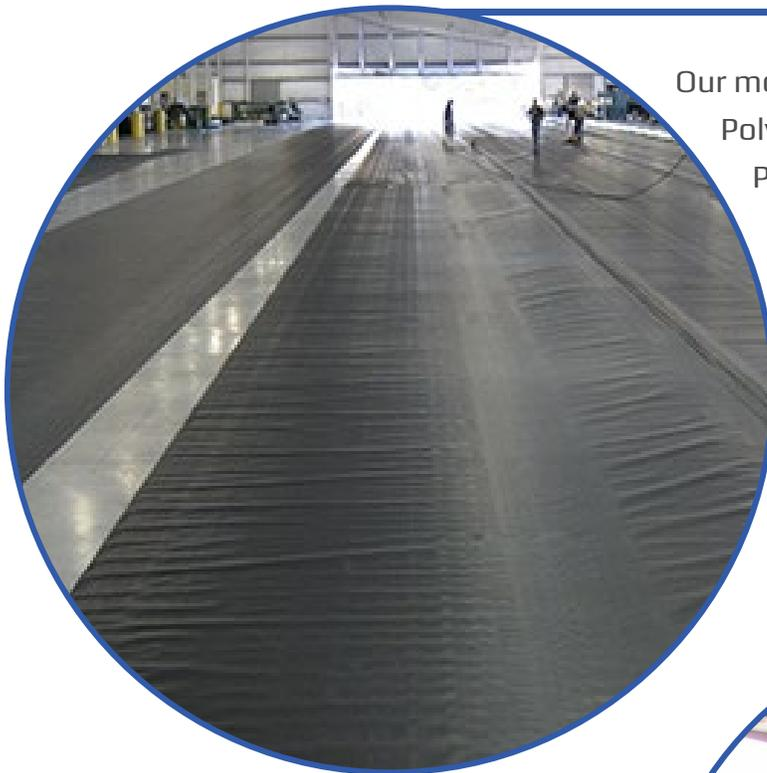
Our most requested liners are HDPE (High Density Polyethylene) and LLDPE (Low Linear Density Polyethylene). Both of these materials can be factory seamed to the size specifications of your project.
