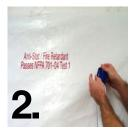
Place and adhere this end at the top of the desired opening. Make sure that the bottom end of the strip aligns to the end of the sheeting you are adhering it to.
