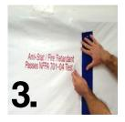
Once adhered, continue to lay and peel the backing off of the zippers as you place the strip onto the sheeting. Gently press it onto the sheeting as you make your way down.
