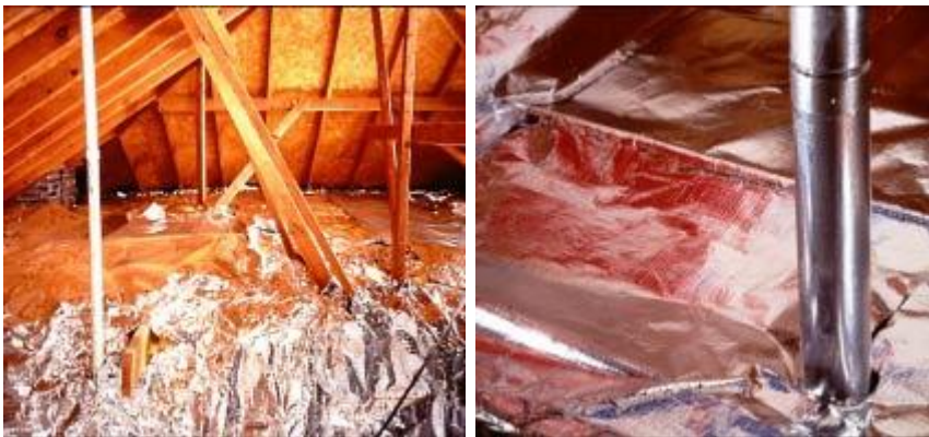
Super R Diamond™ is applied over mass insulation for superior insulating qualities.
