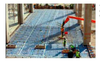
VaporBlock<sup>®</sup> is a high performance underslab vapor barrier designed to retard moisture migration through concrete slabs and concrete walls to protect your structure from:
